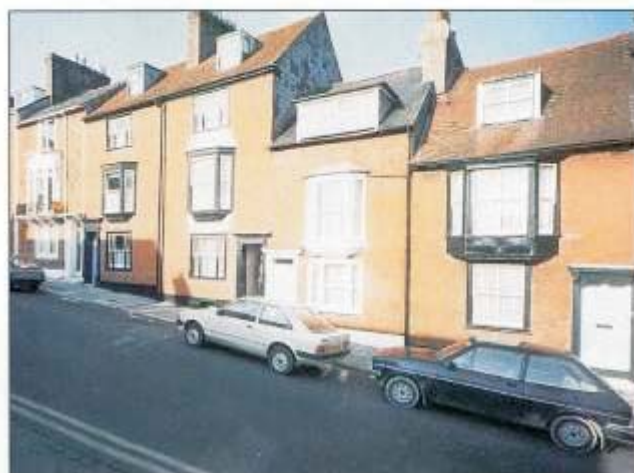
18th century timber and brick terrace, Lewes
