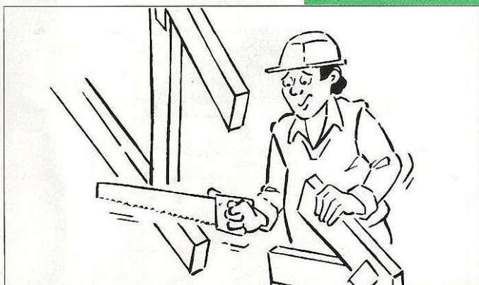
Trussed rafters are designed and fabricated for a particular purpose and to save work. Trusses must not be cut under any circumstance. Truss spacings can usually be adjusted to take hatch openings and chimney breasts. For large chimney breasts, trusses are specially designed and supported. Don't cut or guess, consult your roof truss supplier if you are in doubt.
